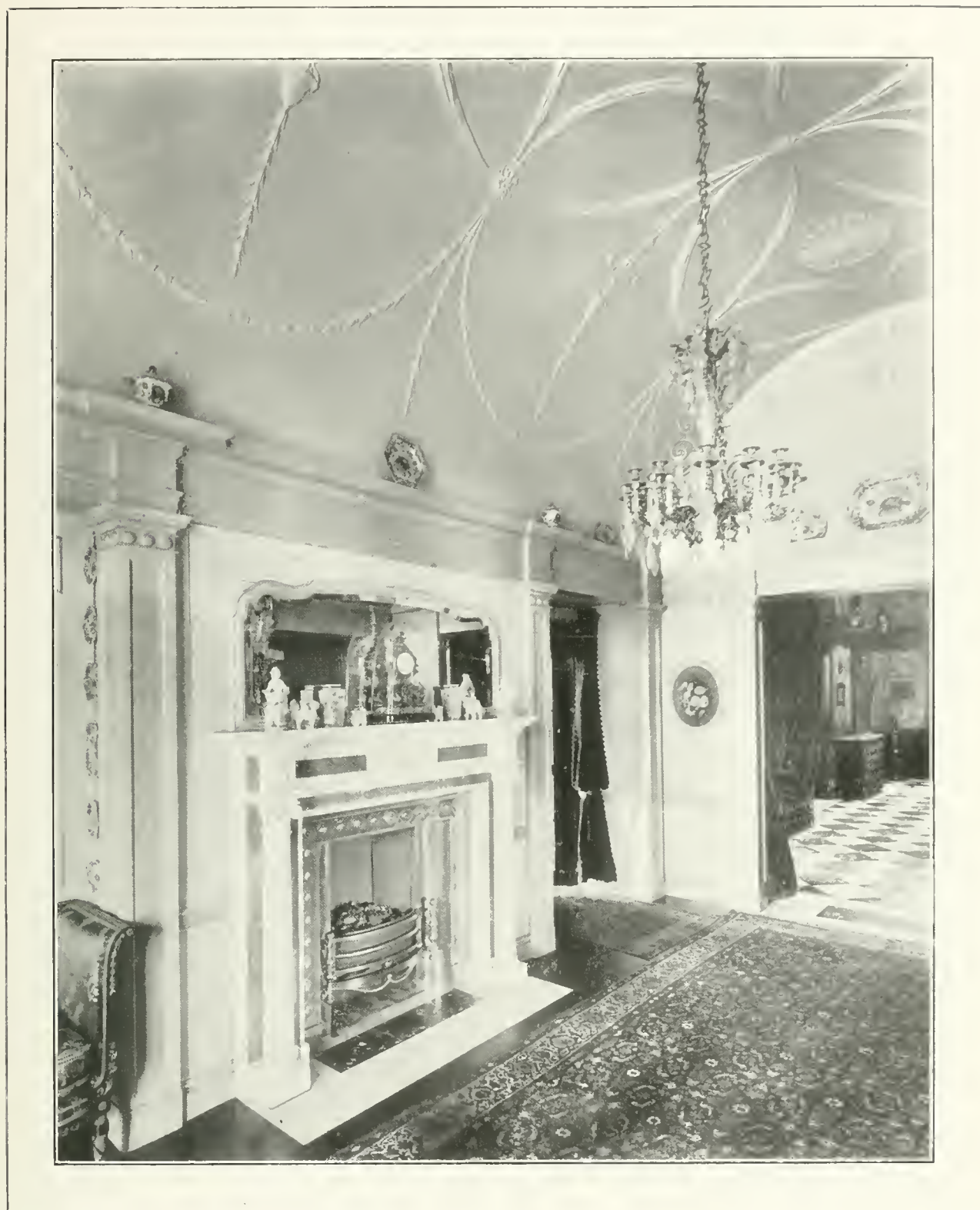
The chimneypiece is of white marble with inlaid bands of coloured marble. The grate is of bright steel. The walls are panelled and painted white, and the barrel-vault ceiling has a simple Adam decoration.
